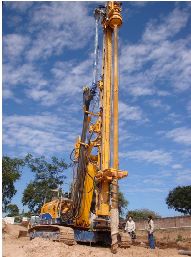
Fig. 4 The FDP pile construction unit
